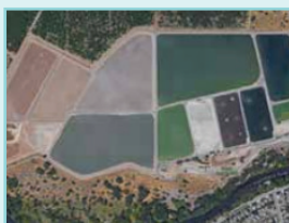
City of Riverbank wastewater treatment plant plan aerial view
