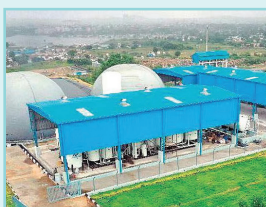
Compressed Biogas Plant (CBG)
