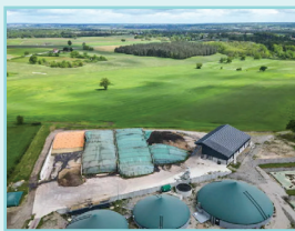
Biomethane injection and anaerobic digestion facility at France
