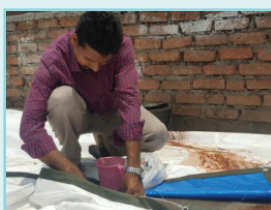
cool roof pilot installation
